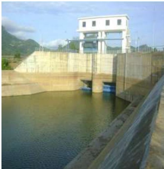
Control Structure Sistem
