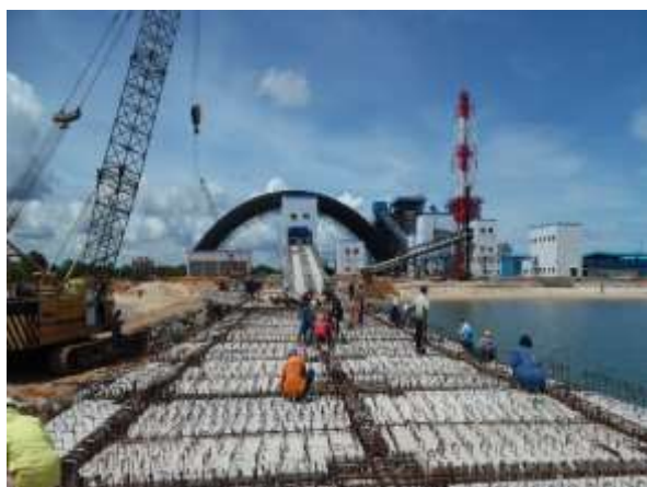
Trestle - rebar installation for slab
