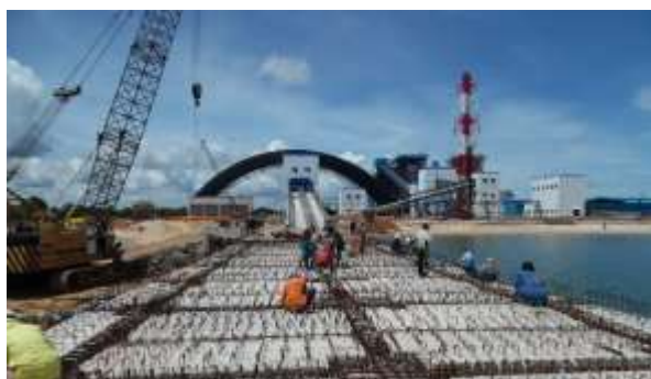
Trestle - rebar installation for slab
