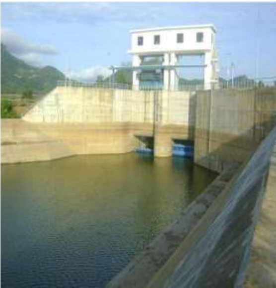
Control Structure Sistem
