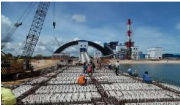
Trestle - rebar installation for slab
