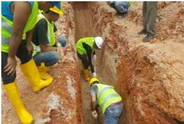
Progress in Site Excavation
