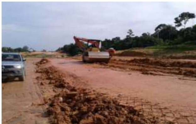
Trial Embankment STA 1+150
