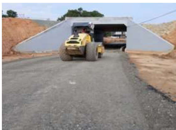
Pemadatan Lokal Road Under Pass Sta 9+998
